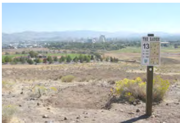
Dirt pad excavated into the ground
