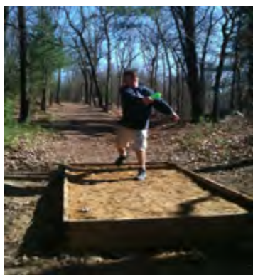
Wood frame filled with gravel
